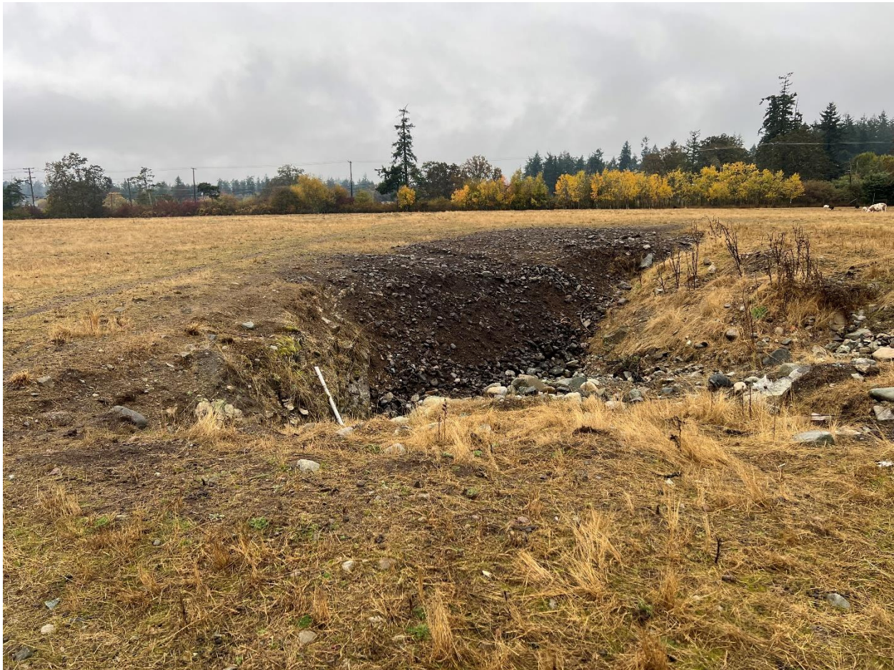
Below Image – Ongoing Restoration of the Northwest Pasture
