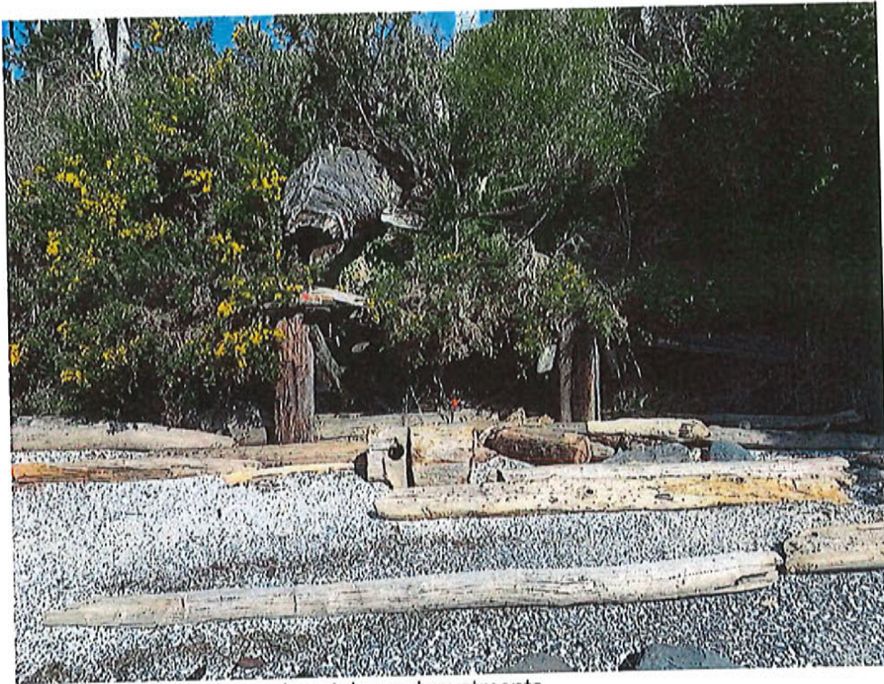
Photo 11. Historical wooden stairs and revetments.
