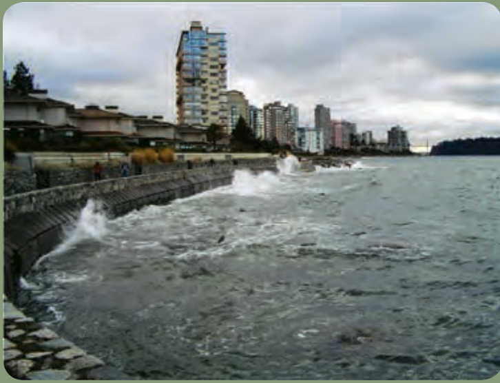
West Vancouver, B.C. Seawall
