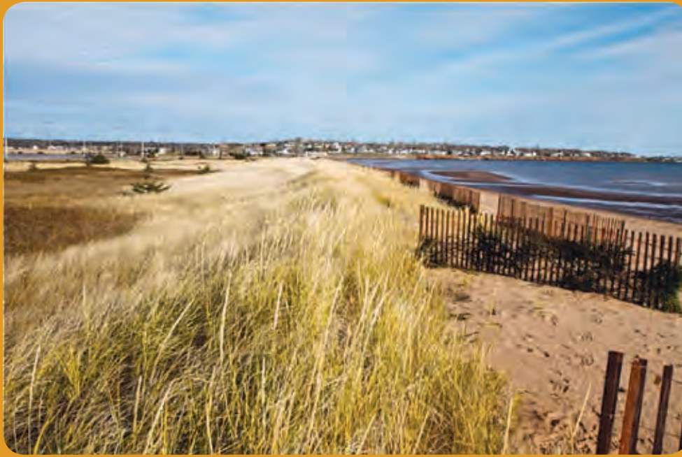
Dune protection consisting of sand fence with spruce boughs, Souris Causeway, P.E.I. (Photo: D. Jardine)
