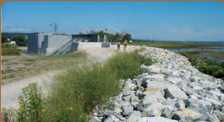
Sea dike and upgraded Oliver Pump Station, Corporation of Delta, B.C. (Photo: Graham Farstad)
